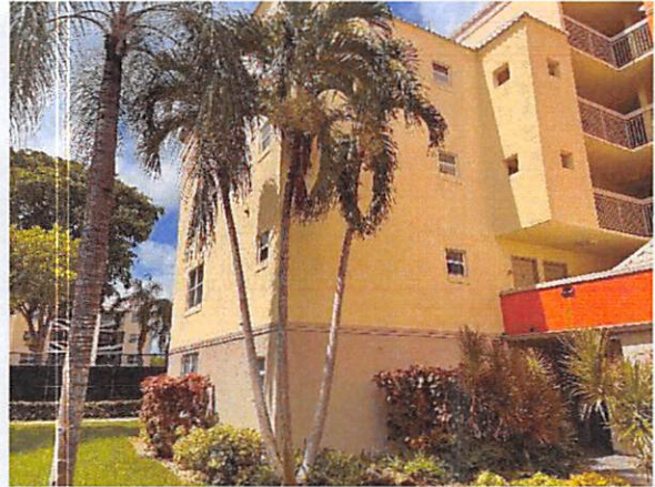
5.a Overall structure in Fair condition
