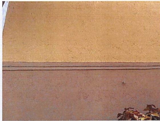
5.e Structure in fair condition
