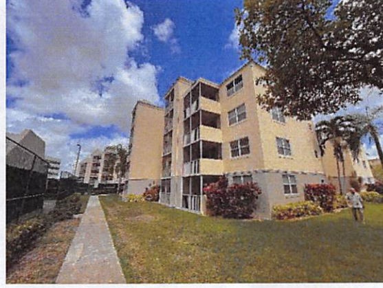
3.b Façade south side
