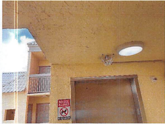
7.b.1 Floor system in fair condition
