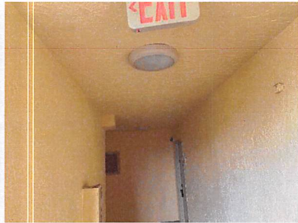
6.k Not rebar corrosion observed.
