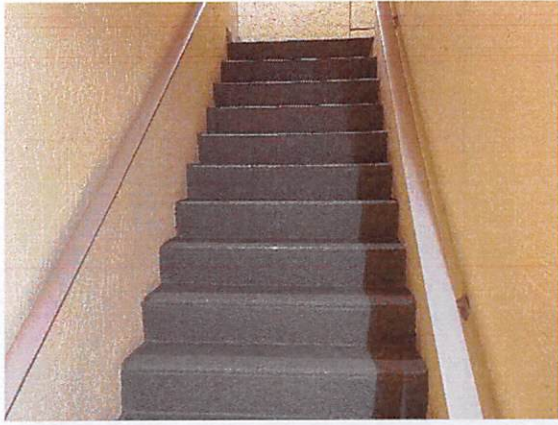
7.b.3 Stair in fair condition
