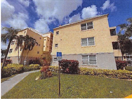
3.b Façade west side
