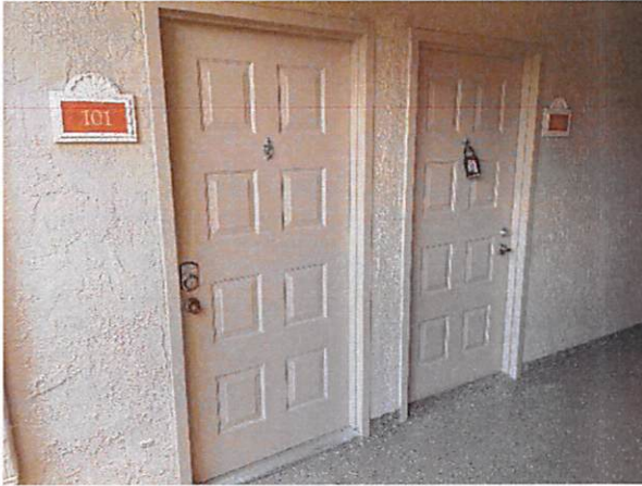
10.c Exterior doors in fair condition
