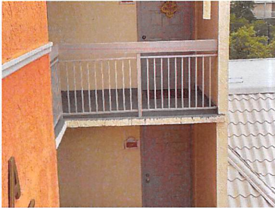
7.b.2 Balconies in fair condition
