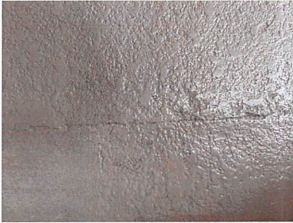
9.b Cracking
