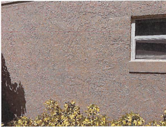
5.f patching on walls
