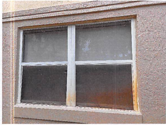
10. Windows in fair condition
