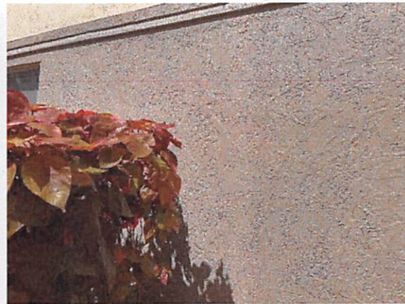
6.a Masonry wall in fair condition
