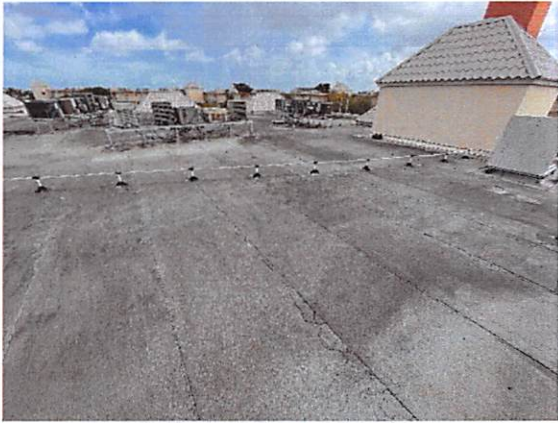
7.a.6 Roof covering in fair condition
