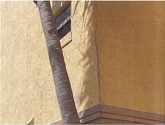
5.b Structure in fair conditions
