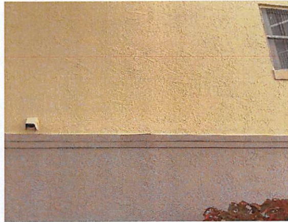
6.a Masonry wall in fair condition
