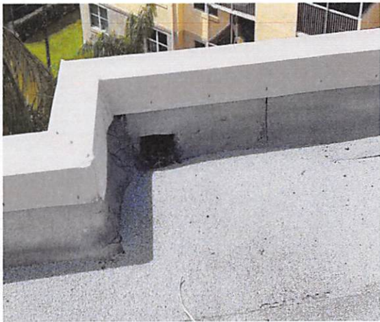
7.a.3 Roof drainage
