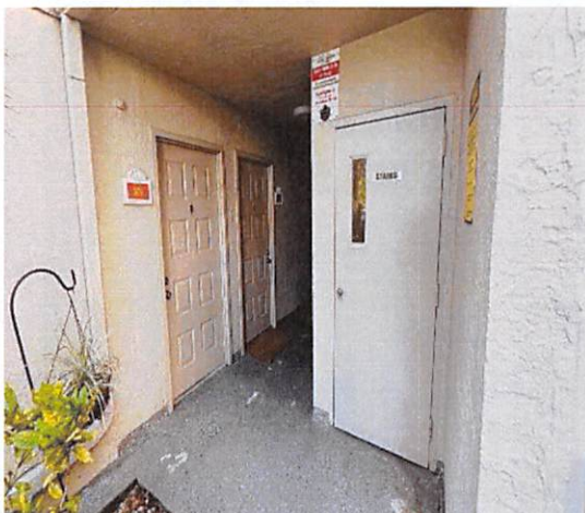
10.c Exterior doors in fair condition
