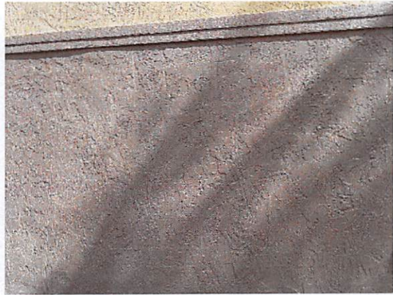
5.e Structure in fair condition
