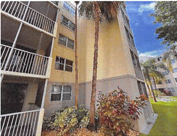
5.b Structure in fair conditions
