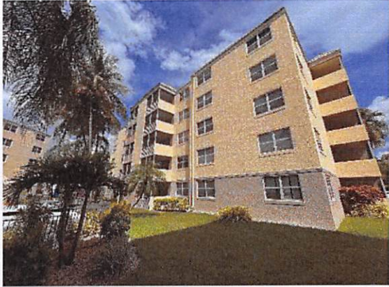
3.b Façade west side
