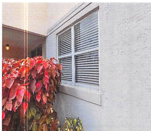
10. Windows in fair condition
