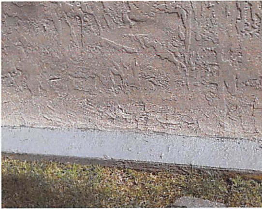
5.f patching on walls
