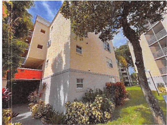
5.a Overall structure in Fair condition
