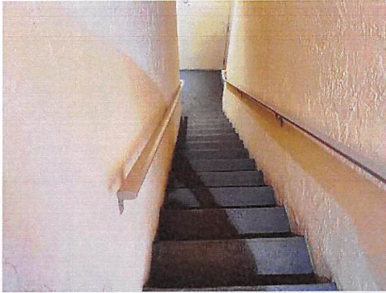
7.b.3 Stair in fair condition
