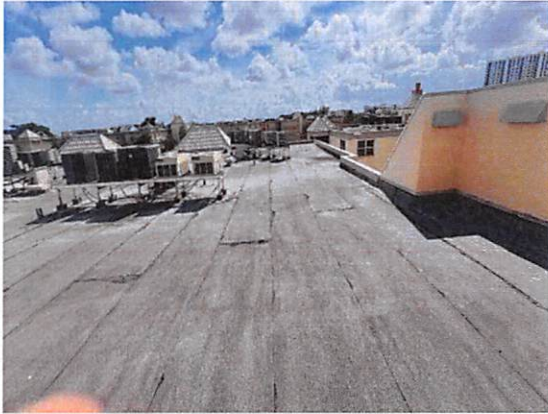
7.a.6 Roof covering in fair condition
