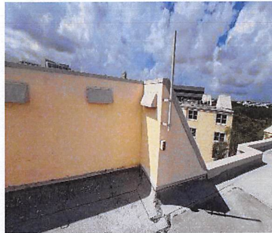
7.a.4 Parapets in fair condition
