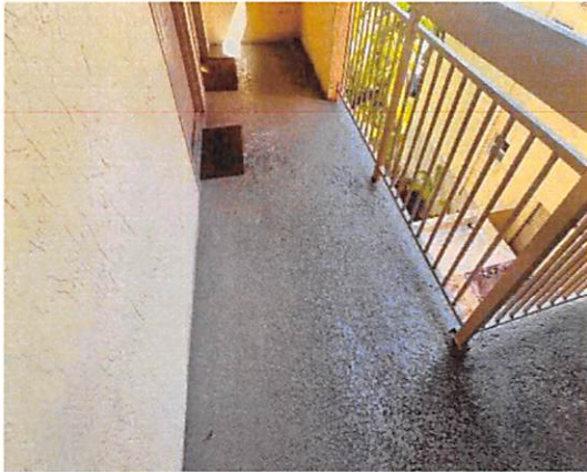
7.b.2 Balconies in fair condition
