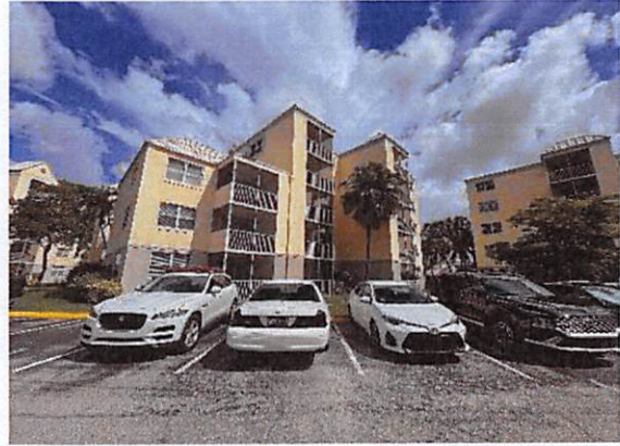
3.b Façade south side
