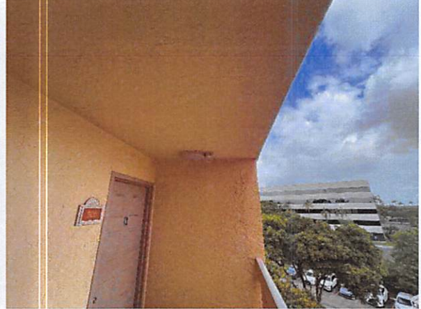
6.k Not rebar corrosion observed.
