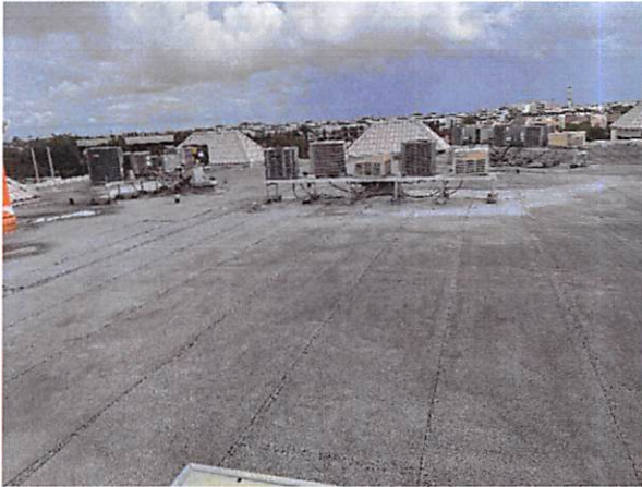
7.a.6 Roof covering in fair condition
