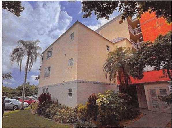
5.e Structure in fair condition
