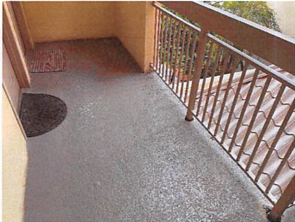
7.b.2 Balconies in fair condition
