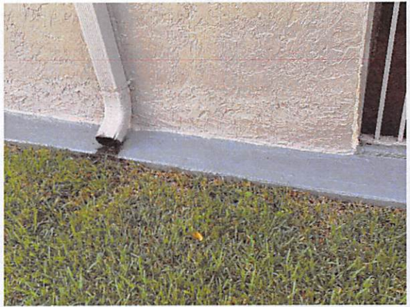
5.f Patching on walls
