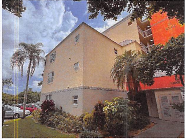
5.a Overall structure in Fair condition
