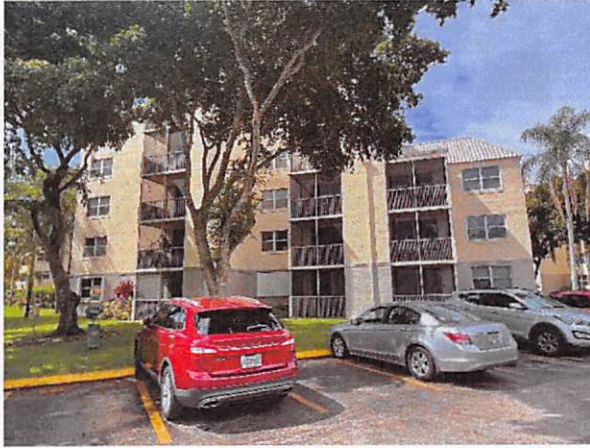
3.b Façade west side
