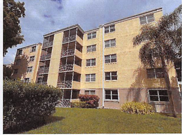
3.b Façade south side
