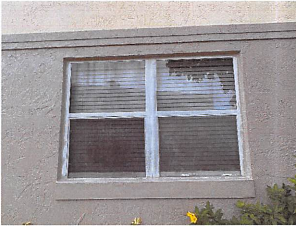
10. Windows in fair condition
