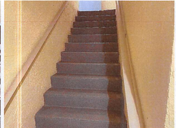
7.b.3 Stairs in fair condition
