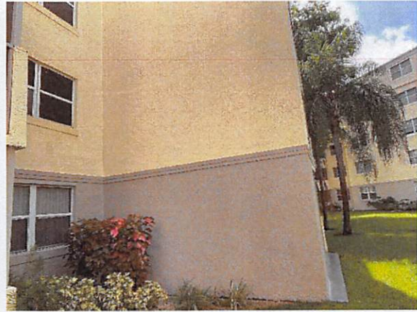
6. Masonry wall in fair condition
