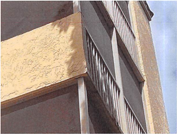
5.b Structure in fair conditions
