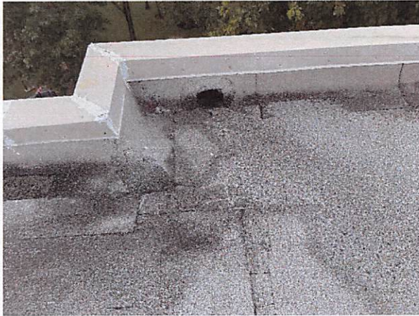
7.a.3 Roof drainage
