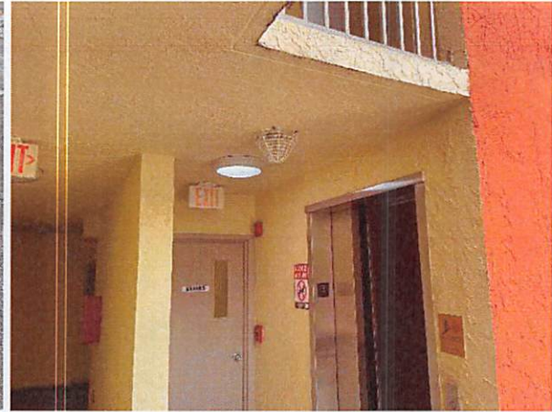
7.b.1 Floor system in fair condition
