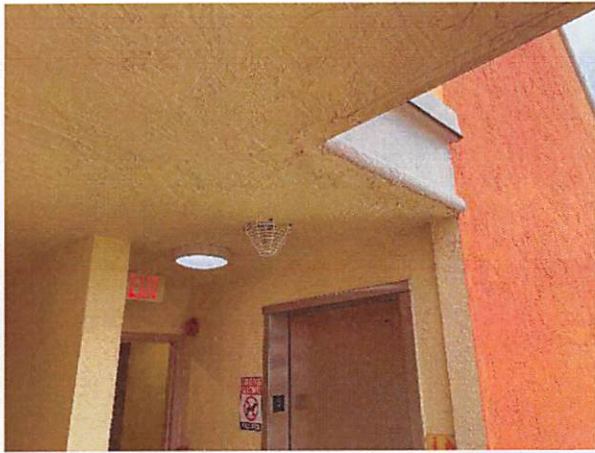
7.a.1 Roof in fair condition.
