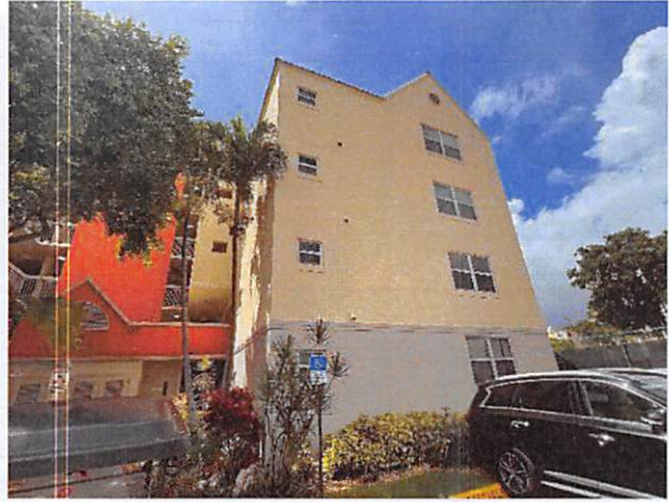
5.a Overall structure in Fair condition
