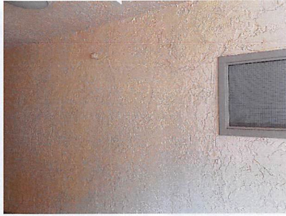
6. Masonry wall in fair condition
