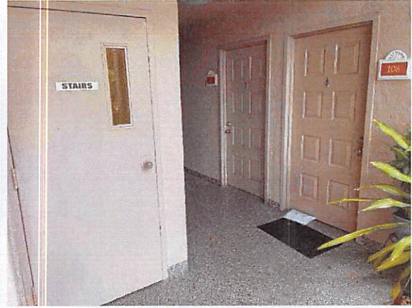
10.c Exterior doors in fair condition
