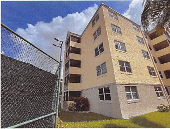
3.b Façade west side
