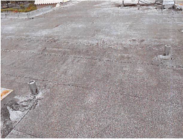
7.a.6 Roof covering in fair condition
