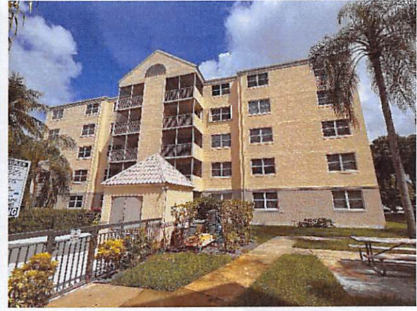
3.b Façade south side
