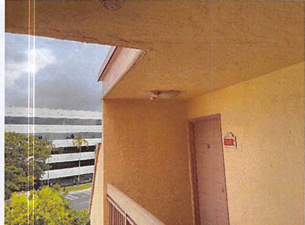
6.k Not rebar corrosion observed.
