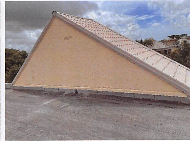
7.a.4 Parapets in fair condition
