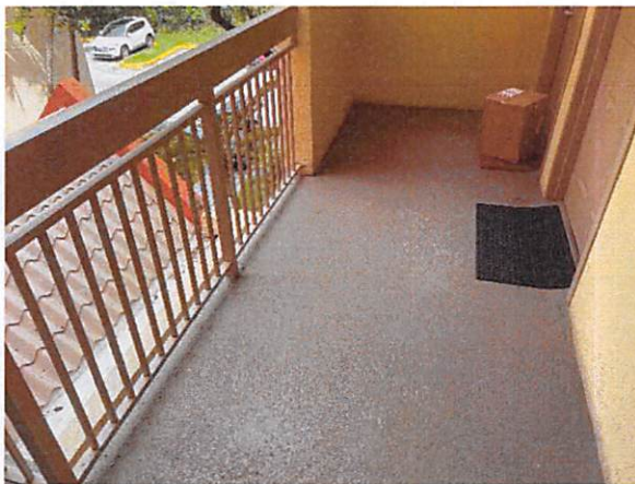
7.b.2 Balconies in fair condition
