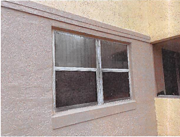
10. Windows in fair condition
