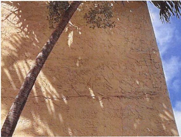
5.f Patching on walls
