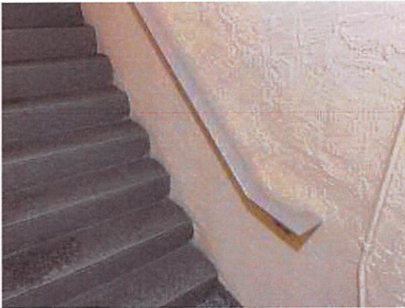
7.b.5 Guard rails in fair condition
