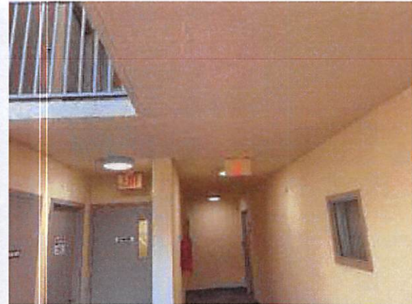
7.b.1 Floor system in fair condition
