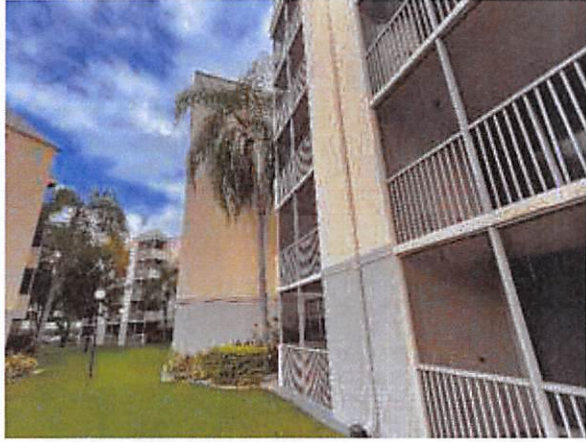
6.f Exterior paint in fair
