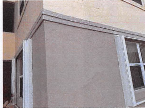
6. Masonry wall in fair condition
