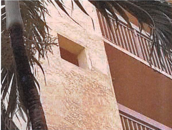
5.b Structure in fair conditions
