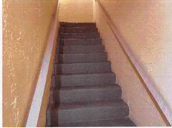
7.b.3 Stair in fair condition
