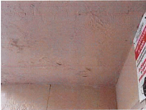
6.j Spalling in small areas.
