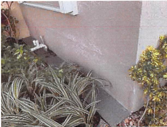
5.f patching on walls
