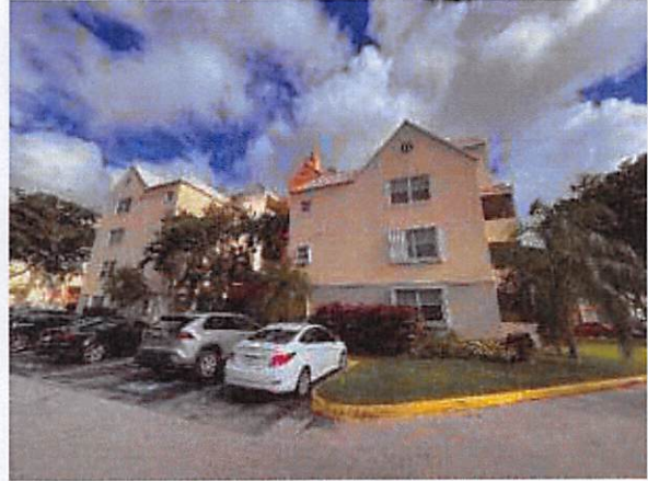
3.b Façade south side
