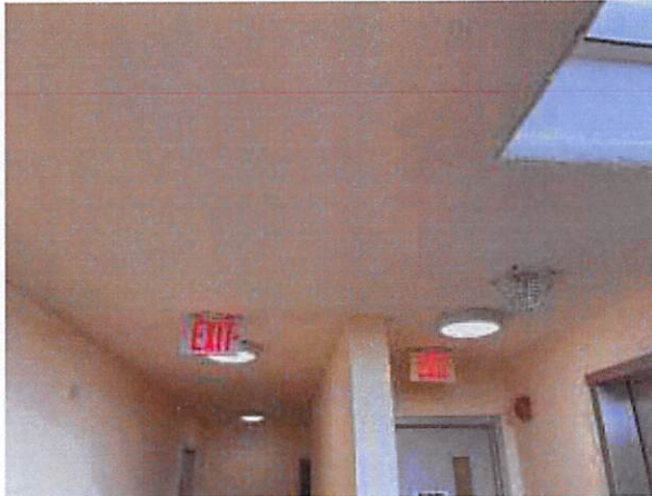
7.a.1 Roof in fair condition.
