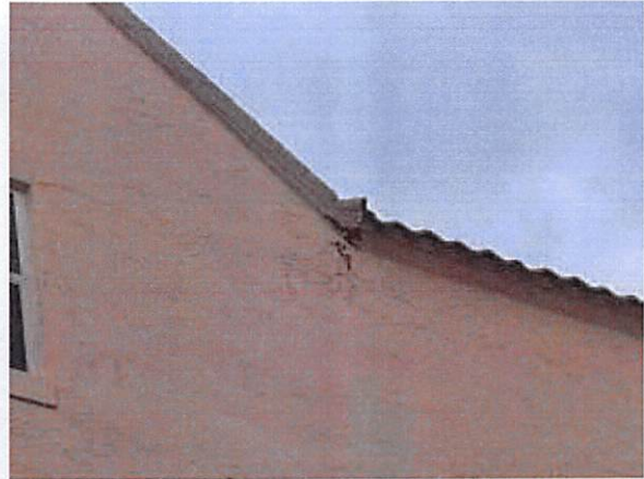
5.e Structure in fair condition
