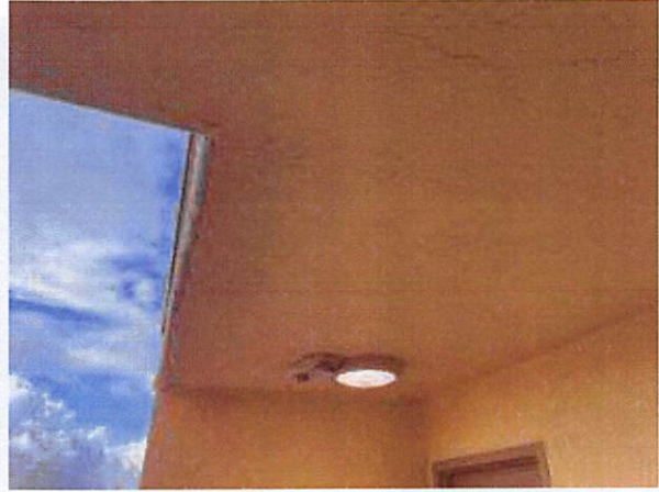
6.k Not rebar corrosion observed.
