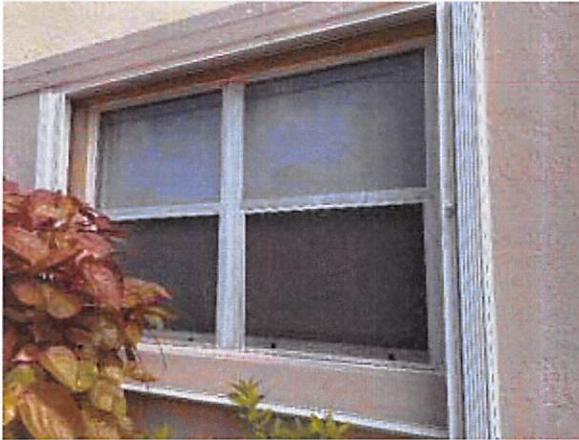
10. Windows in fair condition
