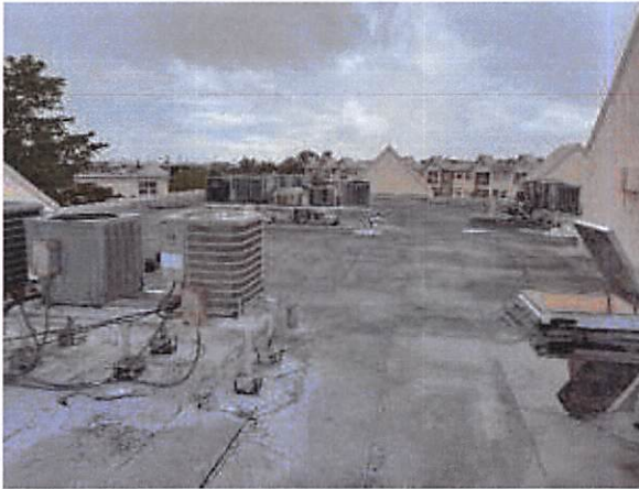
7.a.6 Roof covering in fair condition
