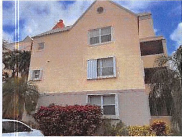
5.a Overall structure in Fair condition
