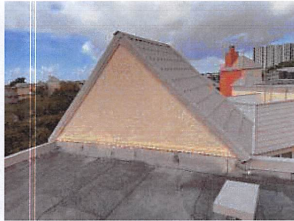
7.a.4 Parapets in fair condition
